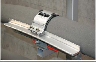
\*Important\*. Do not over tighten the cleat. The liner should be in good firm contact with the cable but does not need to be so tight that the cable bulges at either side of the liner.
