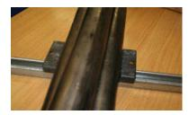
4) Fit the top half of the cleat over the cables. Secure with the M12 setscrews and flange nuts (19mm spanner/socket for setscrews, 16mm spanner/socket for flange nuts).
