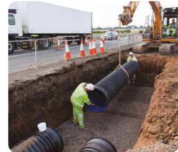
Vital road improvement project relies on Ridgistorm-XL
