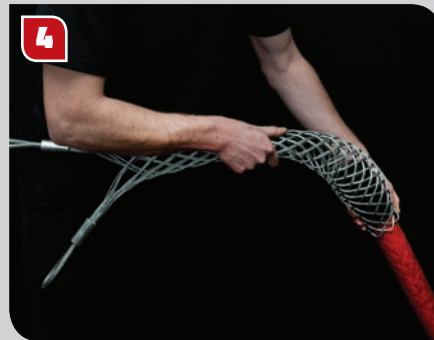
4 ...and pushed over the conductor.
