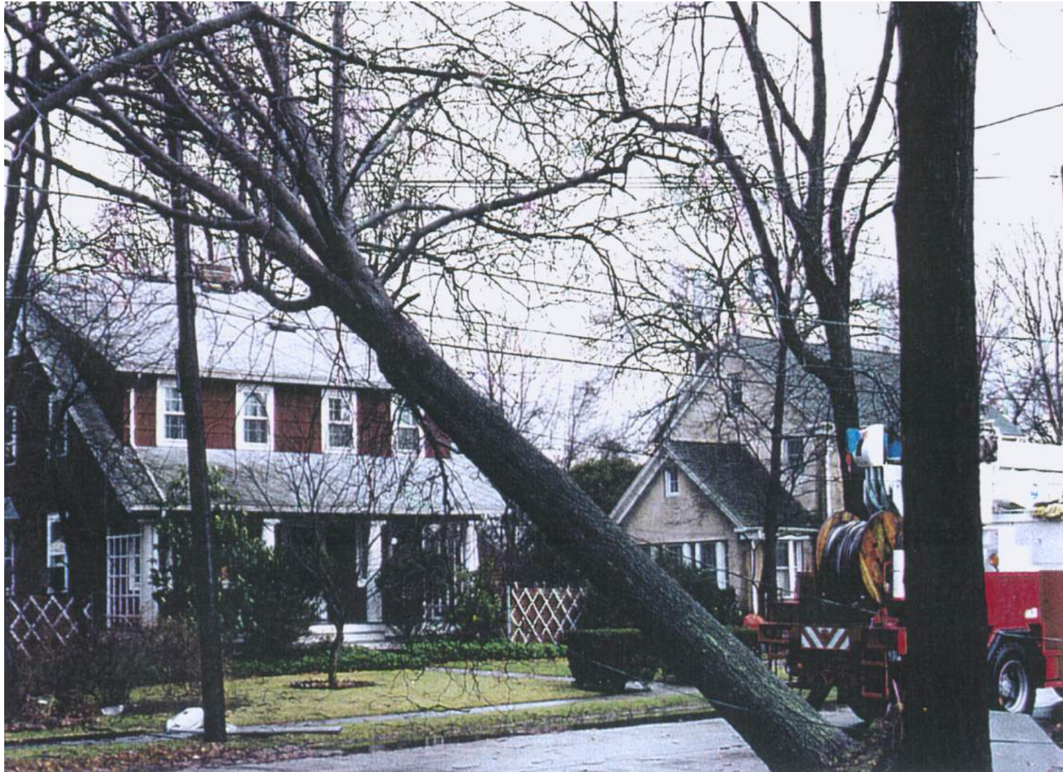
Spacer Cable: Large tree down, line stayed energized
