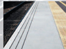
Typical platform construction
