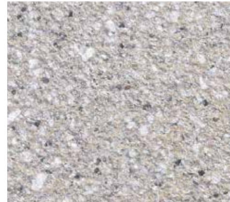
Exposed aggregate finish
