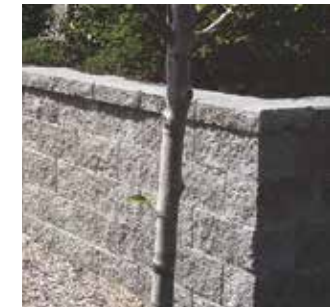
Keystone retaining wall in Flint finish
