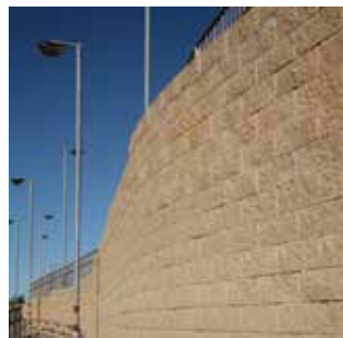
Railway station walls
