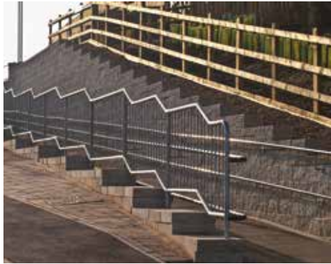
Keystone retaining wall
