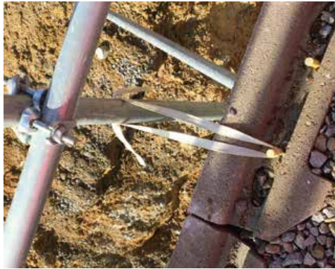
Simple installation of temporary safety railings
