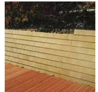
Reinforced earth Slopec
