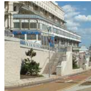
Keystone walls at Southend-on-Sea
