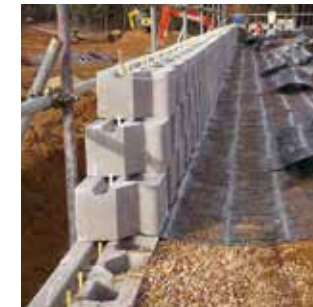
Keystone during construction
