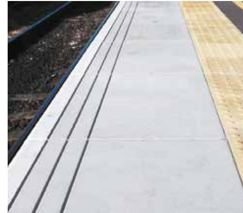
Typical platform construction
