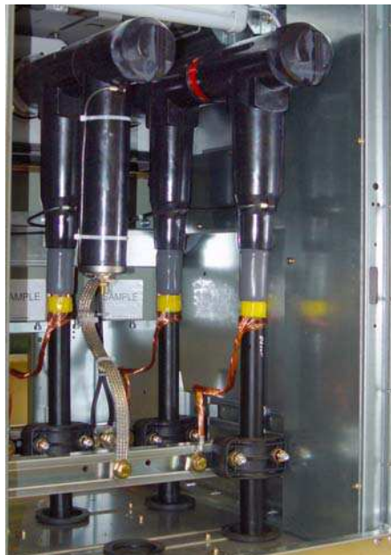
Fig. 99: Mounted surge arrester (example)
