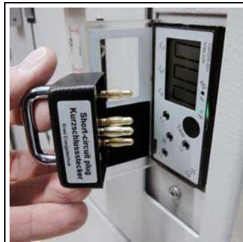
Fig. 116: Short-circuit plug, make Kries, order number 2500029
