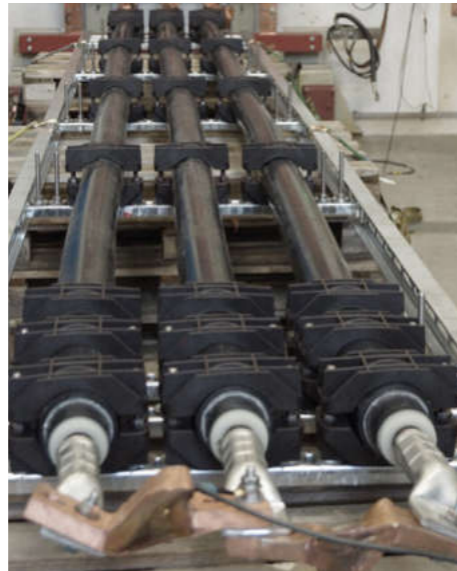
Cable Clamps for single formation after the 1 st test
