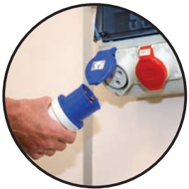
Disconnect all loads.
