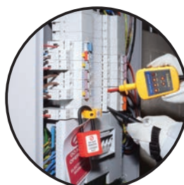
Test the supply is isolated.
