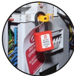
Isolate the source of supply. Lock off and place warning signs.
